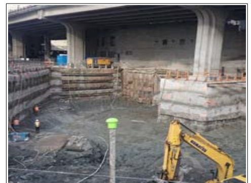
Pic 2: Construction site
